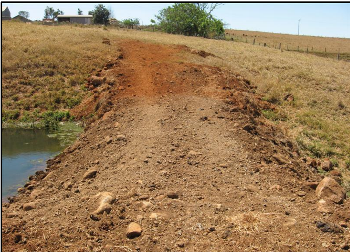
Figure 21. Sediment retention dam below paddock traps sediment and prevents it entering waterways.
