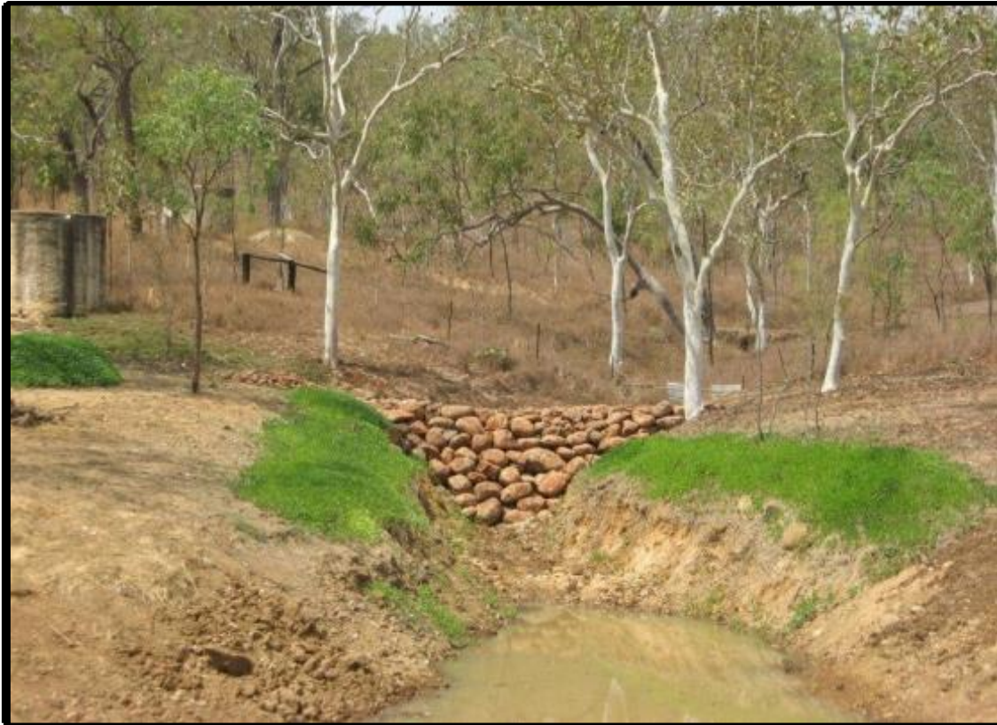
Figure 20. Sediment retention dam with rock wall to reduce water velocity and trap sediment.
