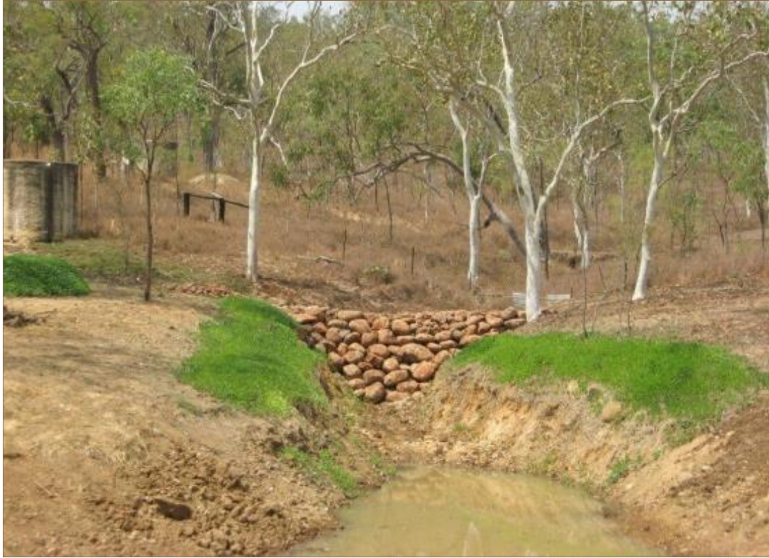
Figure 20. Sediment retention dam with rock wall to reduce water velocity and trap sediment.
